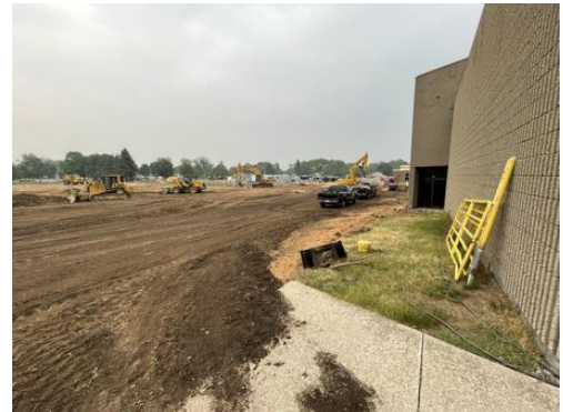
Site Work Near Auditorium
