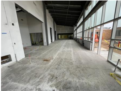
HS Office Entry
