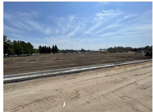
Site Work Near Bus Loop
