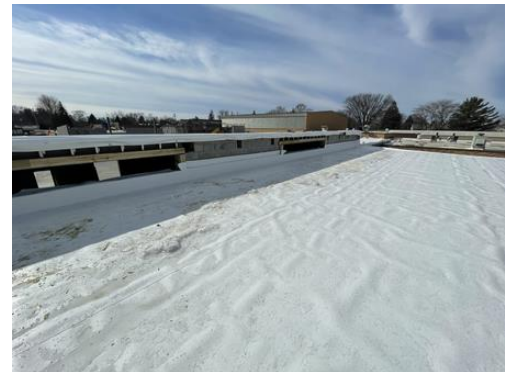
HS Classroom Roof
