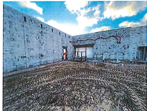
MS Office Addition
