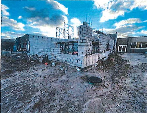
MS office Addition
