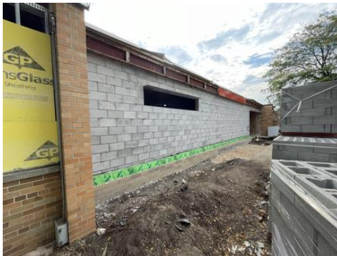
New Lockerroom Exterior Wall
