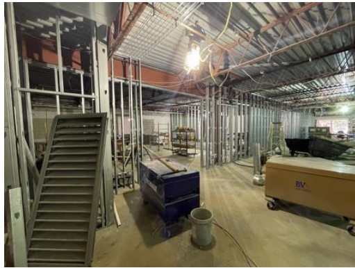
MS Servery / Cafeteria Walls
