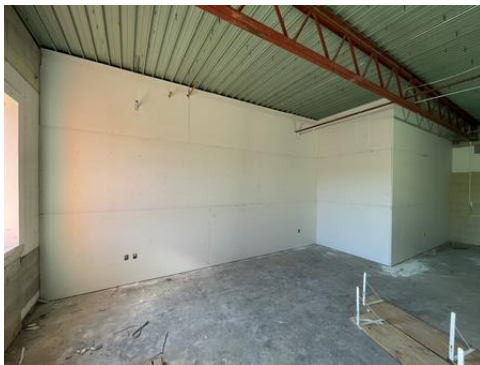
MS Classroom Partition Wall
