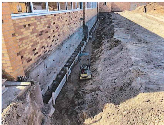
HS office Footing Tie In
