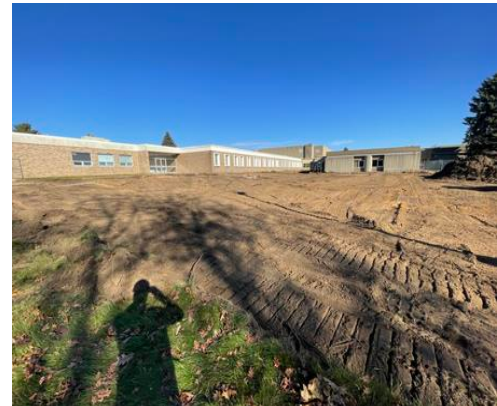
Prep Work for MS Addition
