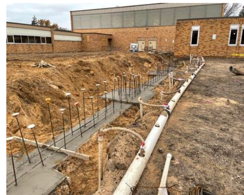
Dewatering in Place for Foundations
