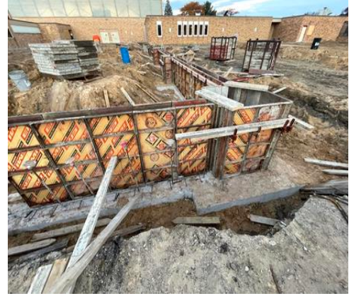
Foundation Wall at Office
