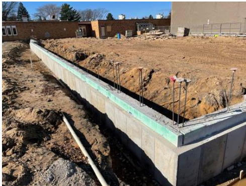
Classroom Addition Foundation Wall
