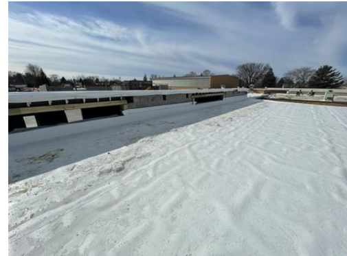
HS Classroom Roof
