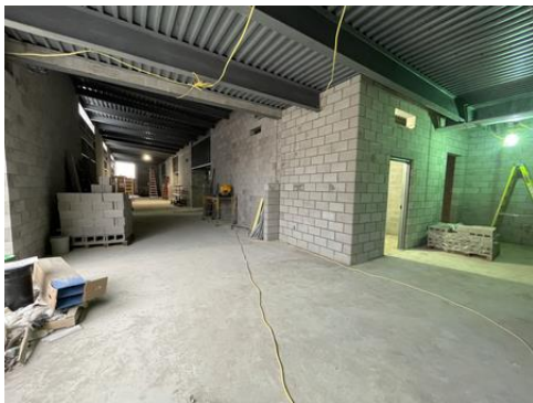
HS Classroom Hallway
