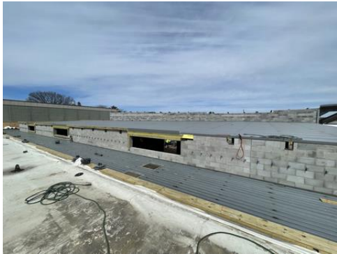
HS Office Roof
