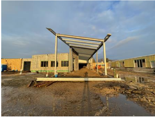
HS Office Addition
