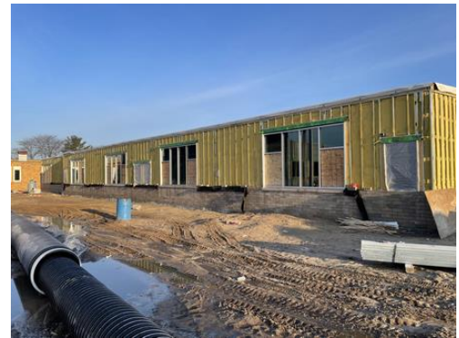
HS Classroom Windows Installed
