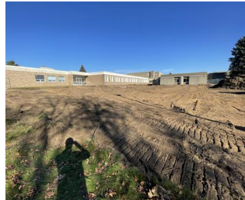
Prep Work for MS Addition
