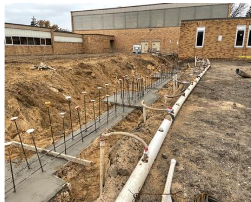
Dewatering in Place for Foundations
