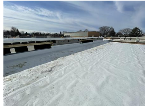
HS Classroom Roof
