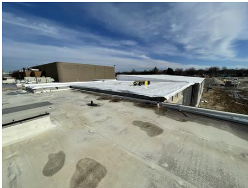
HS Classroom Roof
