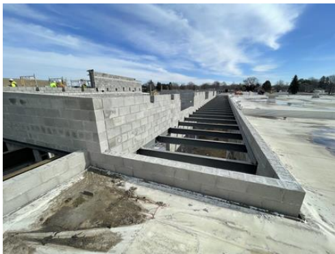
HS Office Steel Framing
