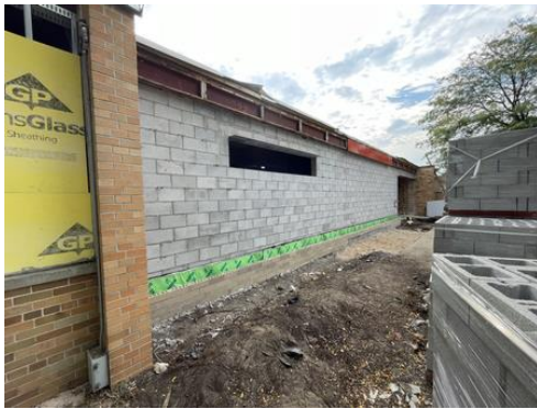
New Lockerroom Exterior Wall
