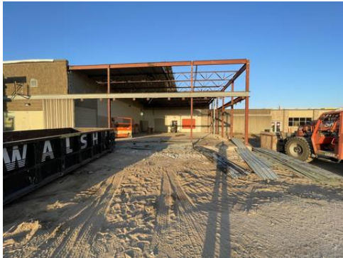
MS Building Demo
