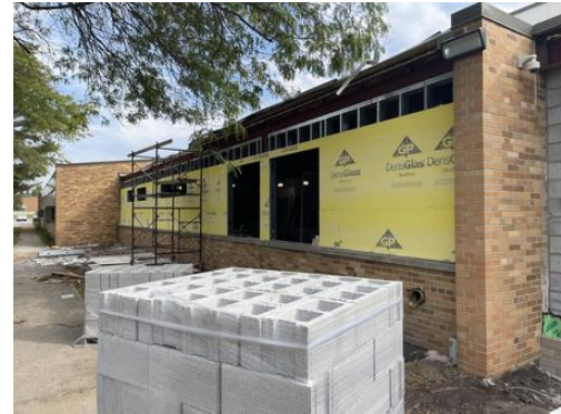
New Lockerroom Exterior Wall
