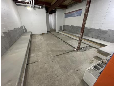
HS Locker Room
