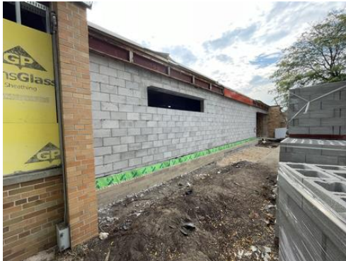
New Lockerroom Exterior Wall
