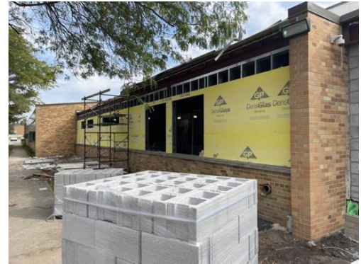
New Lockerroom Exterior Wall
