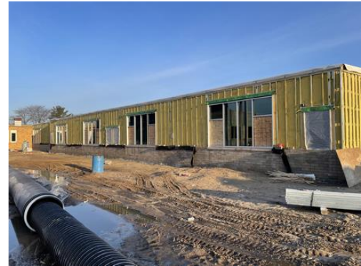
HS Classroom Windows Installed
