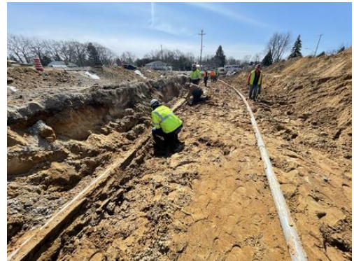
HS Electrical Relocation
