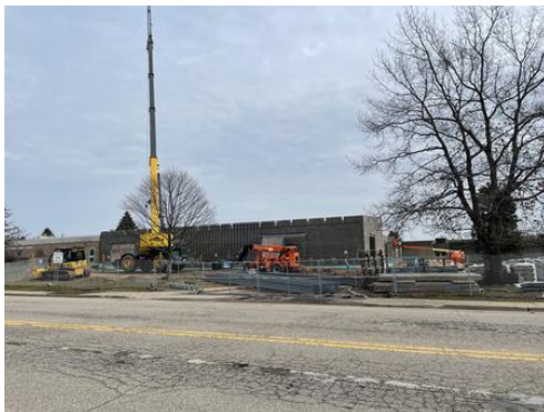
MS Classroom Exterior
