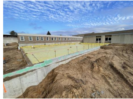
MS Floor Prepped
