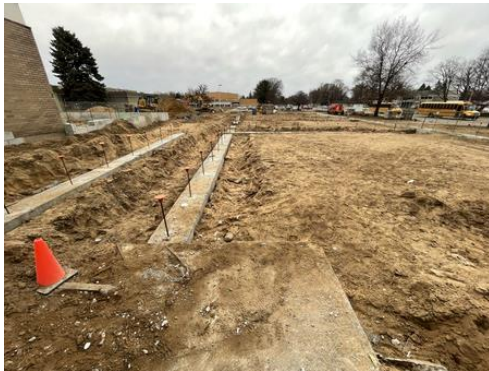
Interior footings in MS Classrooms
